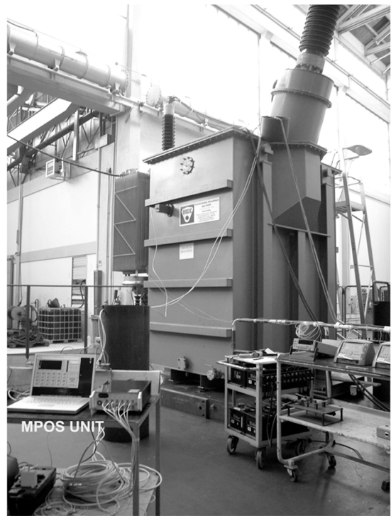
Fig. 7. Photo of the 20 MVA, 345/√3 kV-20 kV (CORE type) power transformer and the MPOS unit at laboratory test facility.
